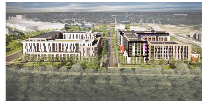
The view from Shingle Creek Parkway, looking east into the heart of the Phase 1 site
