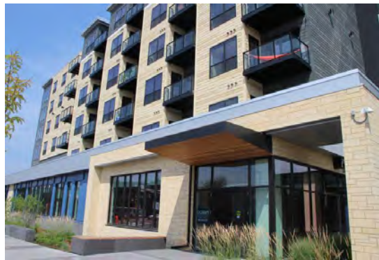
Columbia Heights City Hall integrated with new mixed-use development.
